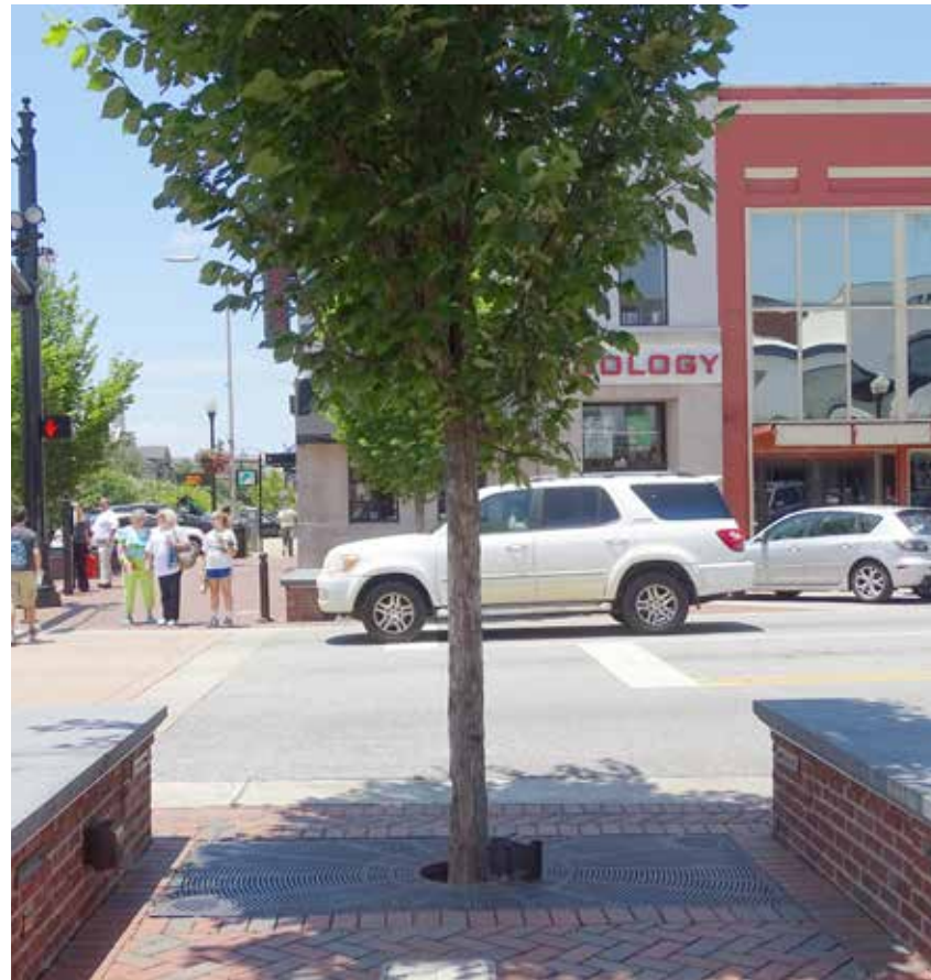
Trees planted with permeable pavers can filter more runoff and grow better..
