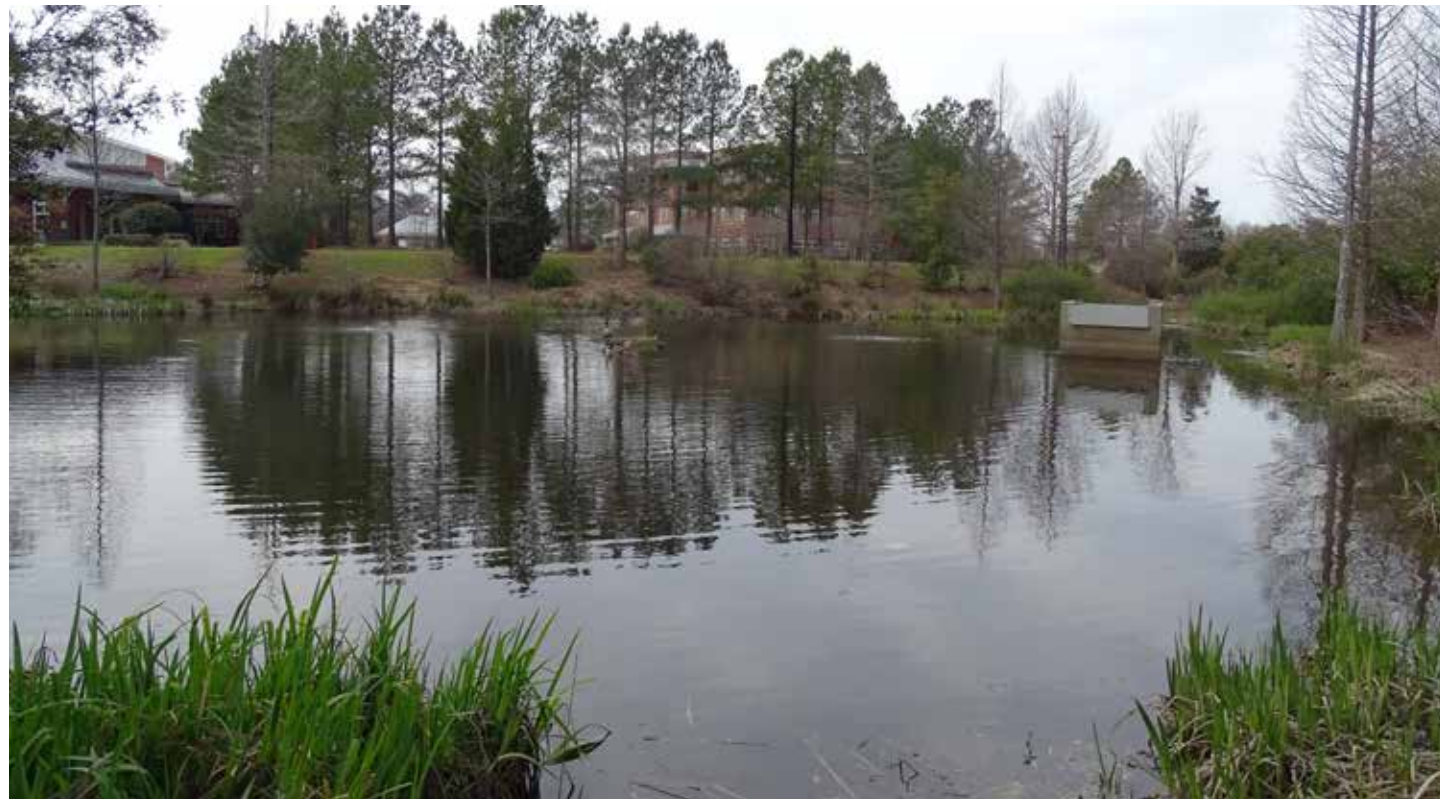
Vegetated stormwater pond helps detain and clean runoff..
